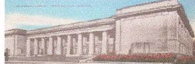
Cropsey Auditorium City Library 914 Pennsylvania Ave
